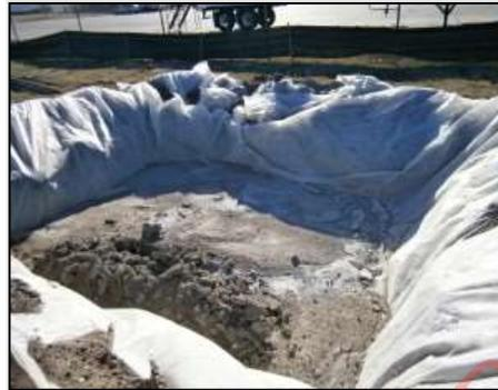
Plate 3-1 Typical concrete chute wash out areas
